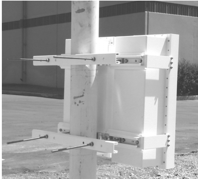
Figure D-4. Rear View of Converters Installed on Pole
