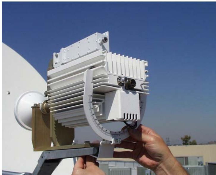
Figure C-6. Installing the SSPA
