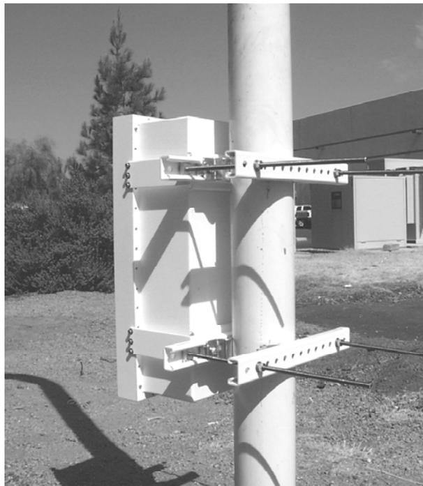
**Figure 6-4. Rear View of Converter Installed
