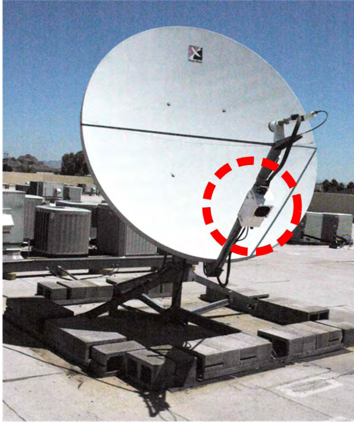
Figure 5-12. Spar Mount Installation Example
